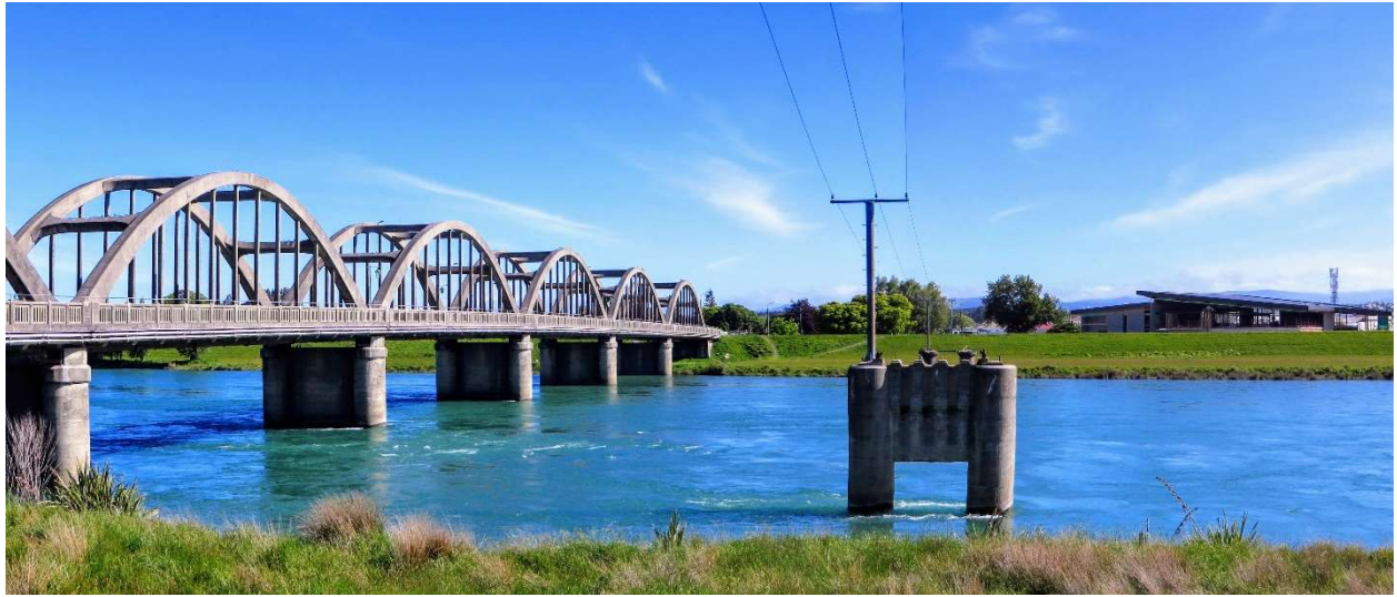
Balclutha bridge, 11,000 volt Clutha River crossing & new Community Hub
