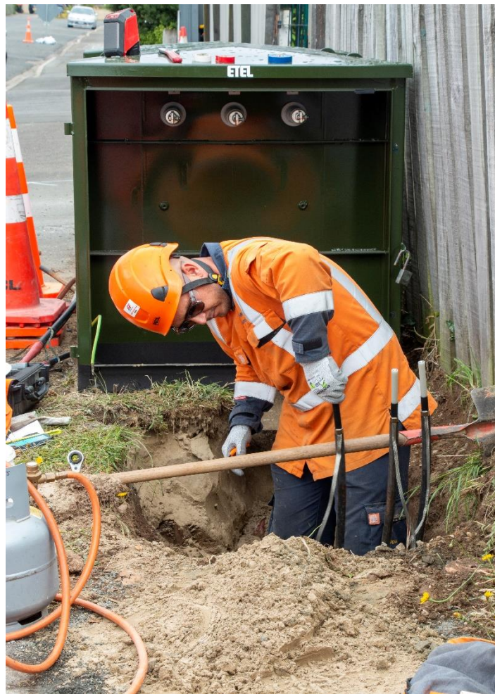
A transformer replacement in Rodney Street, Invercargill
