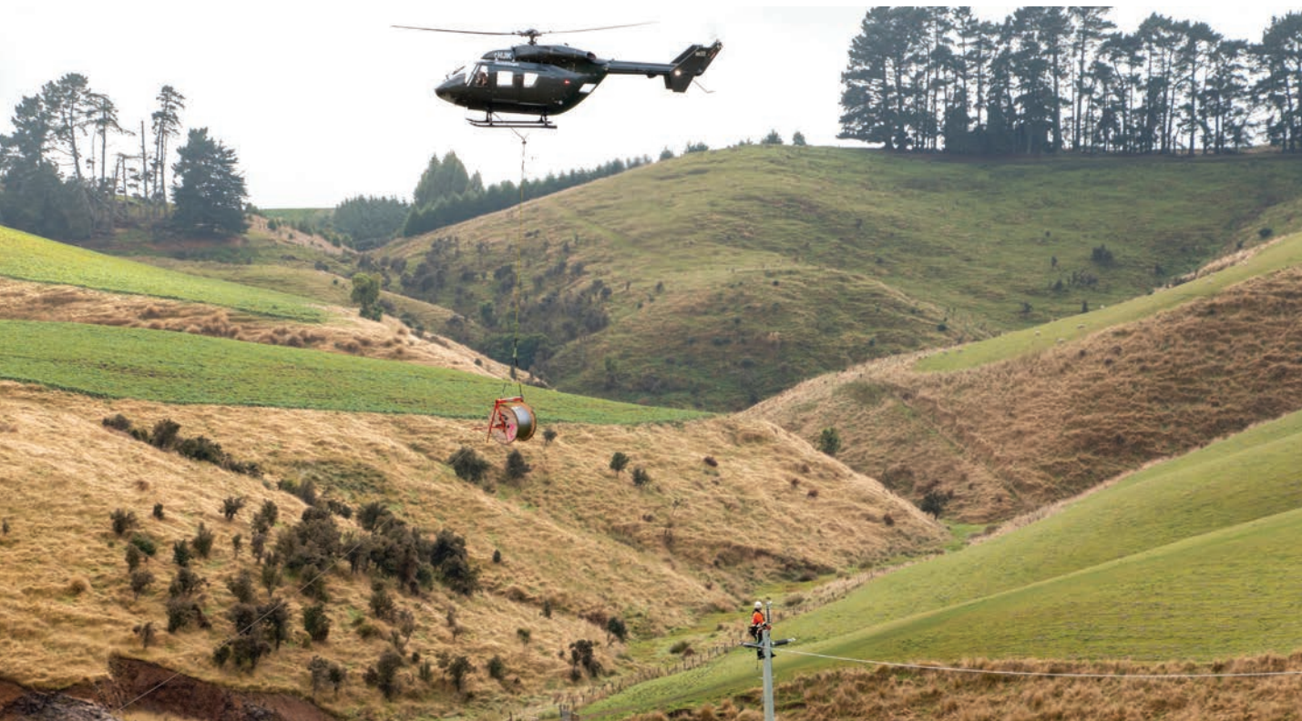
33kV Conductor installation at Kaiwera Downs Wind Farm.
