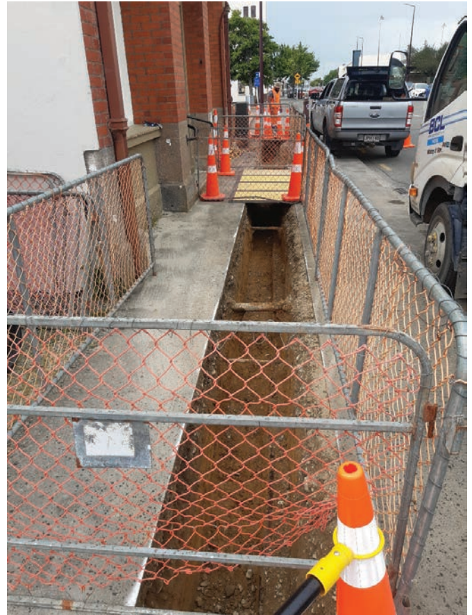
Cable replacement Esk Street, Invercargill.
