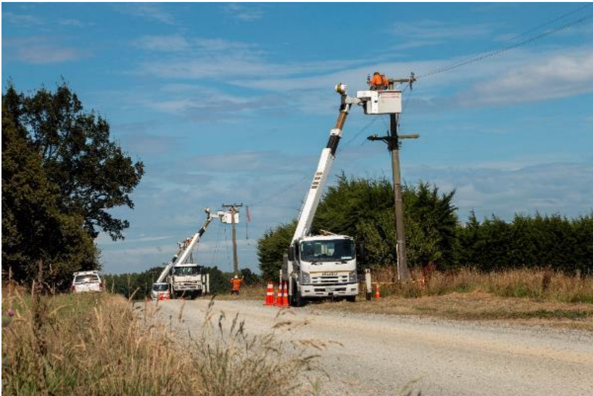
11 kV Line Rebuild - Calder Road, Centre Bush
