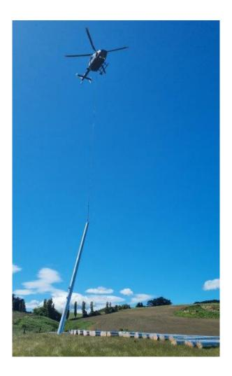
A helicopter transporting one of the 179 poles to site during the construction of the 33kV line linking Mercury NZ's new Kaiwera Downs wind farm to The Power Company Ltd network in Gore.
