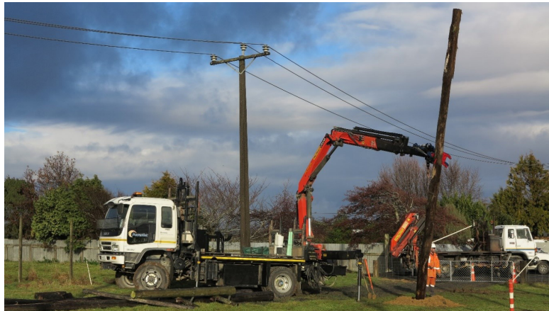
The pole grab at work.
