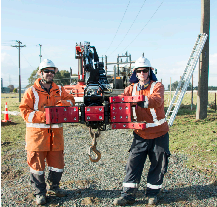
PowerNet line mechanics with the pole grab.
