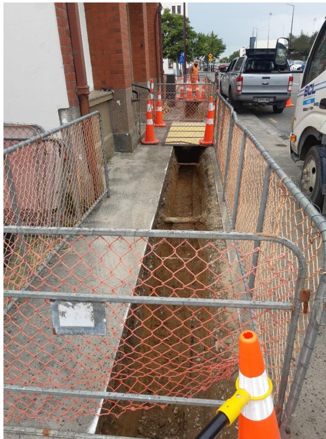
Fault repairs in Esk Street, Invercargill
