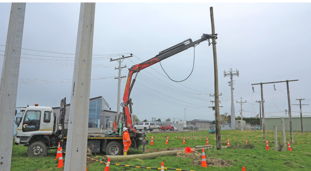
The pole grab at work.
