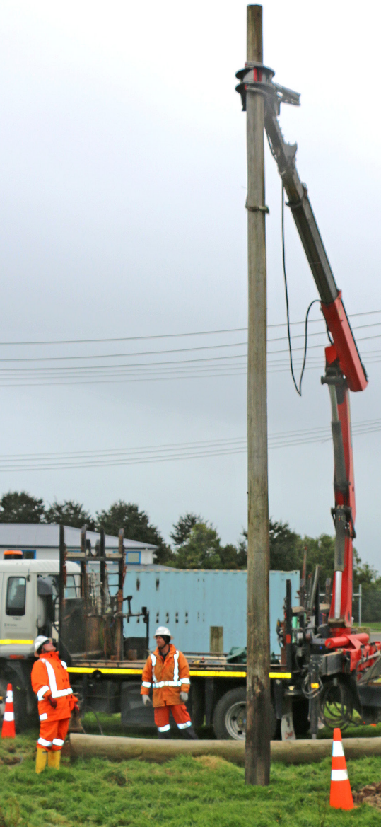
The pole grab in action.
